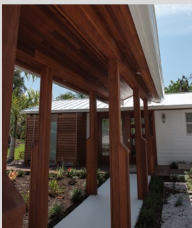
Ipe Soffits & Posts
